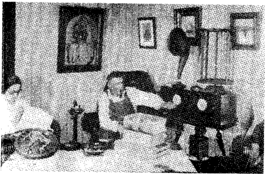
A GE receiver of 1923 being used by a farm family. Note rotative loop antenna and goose neck speaker which could be plugged into different audio stages.
